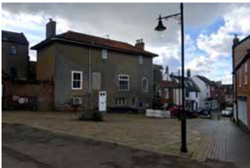
Church Approach before
