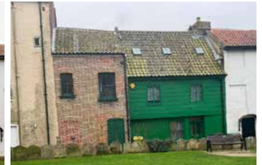
39 Market Place after (rear view)
